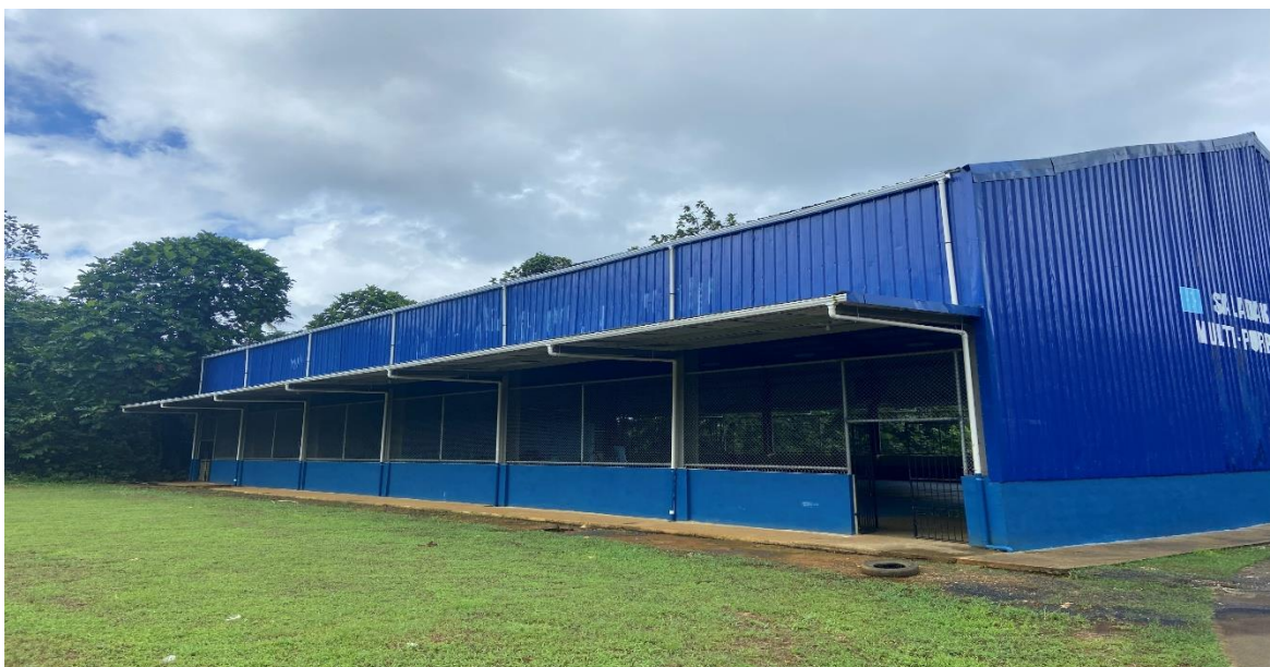
Left Side of Gymnasium
