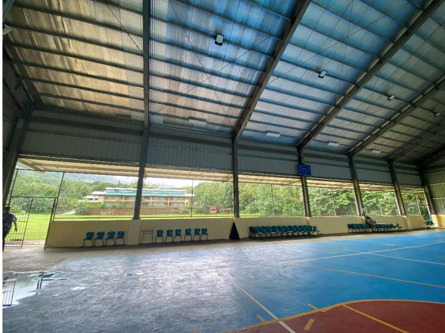
Left Side of Gymnasium
