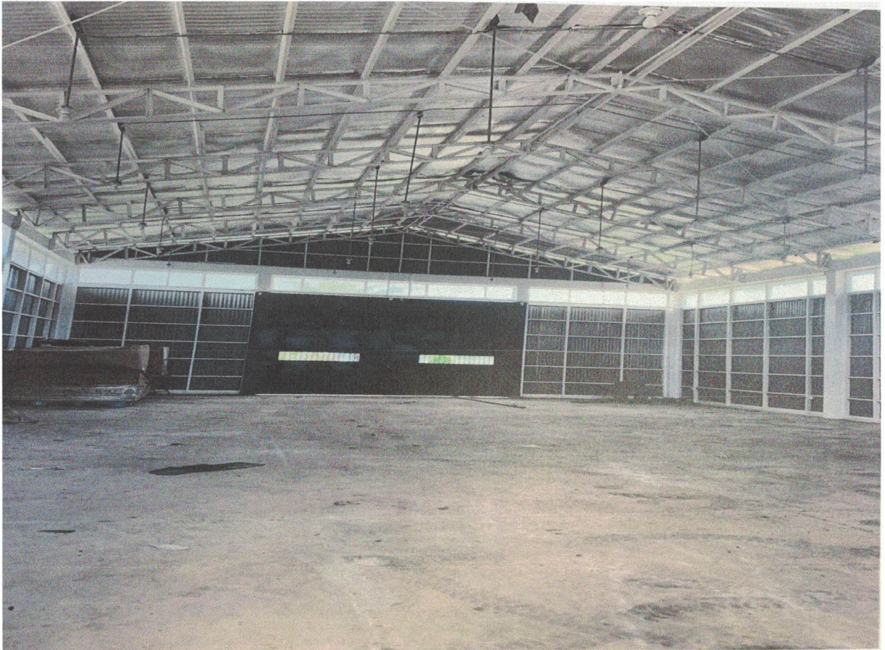
Exhibit II Inside of the Facility
