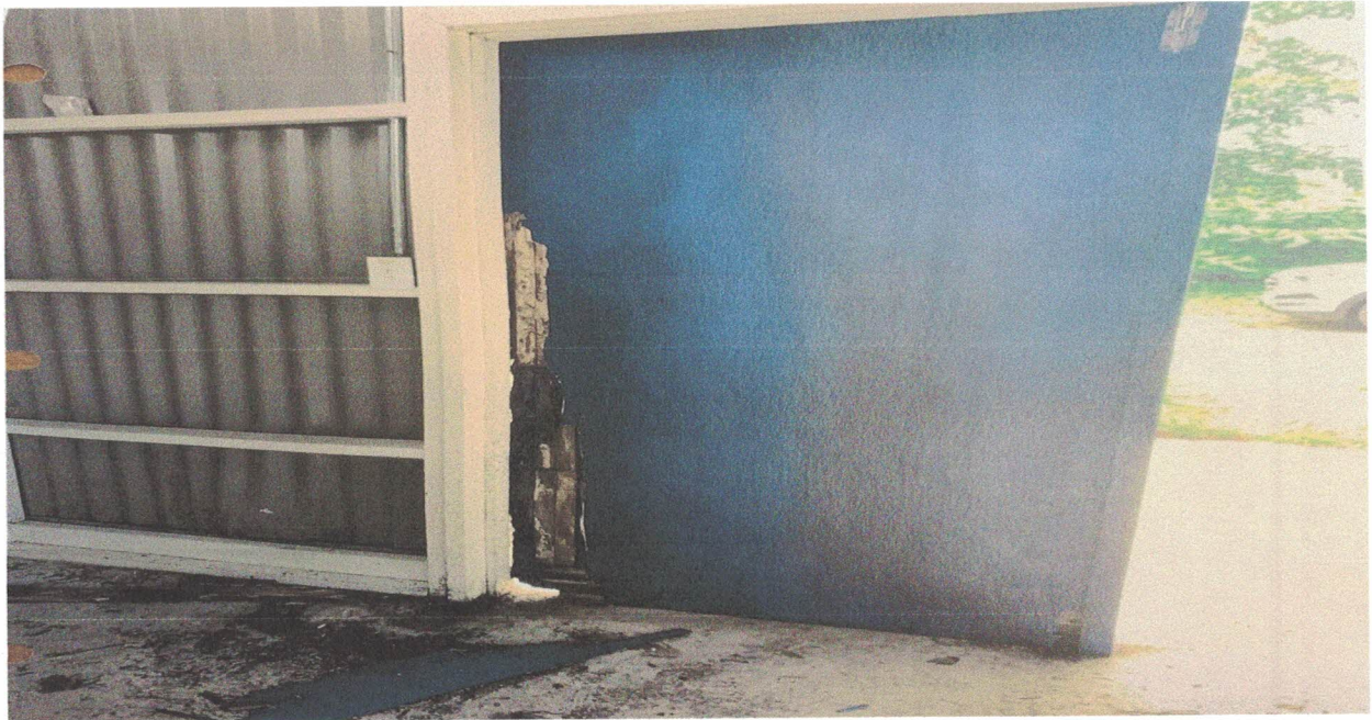
Exhibit I Front door inside of the New Recycling Facility
